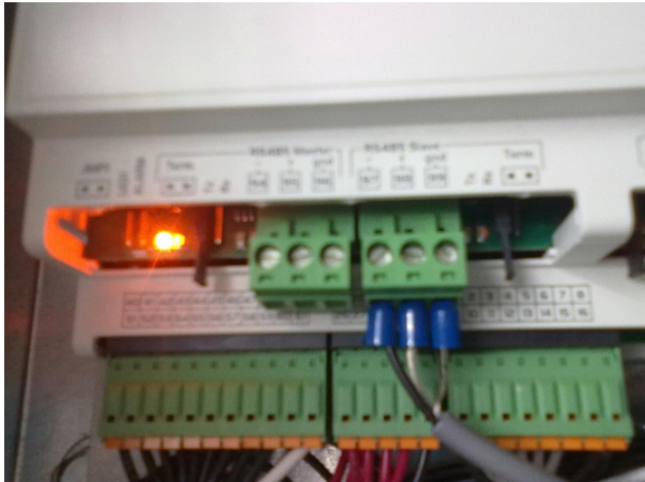
Multi-Zone Leak Detector Wiring
